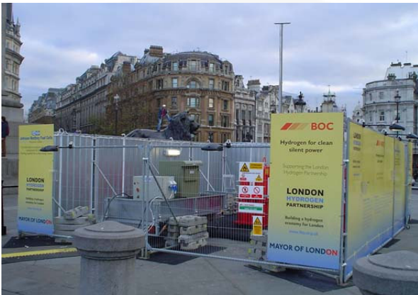
Fuel cell and Hydrogen gas compound.
