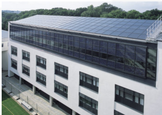
UEA Zuckerman Institute building-integrated PV array.
