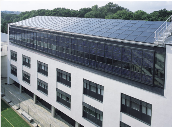
ZICER building (© BP Solar)
