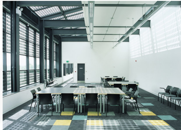
Exhibition hall shading provided by PV (© BP Solar)
